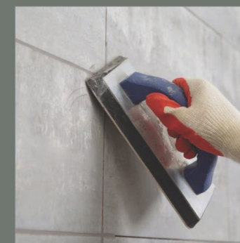
Joint Grouting
