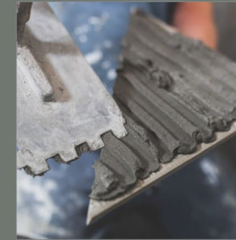
Cement Laying On Tile
