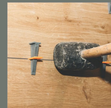
Remove Wedges Ones It Dry
