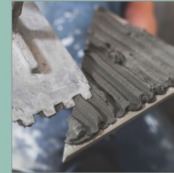
Cement Laying On Tile
