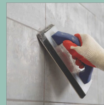
Joint Grouting
