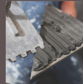
Cement Laying On Tile
